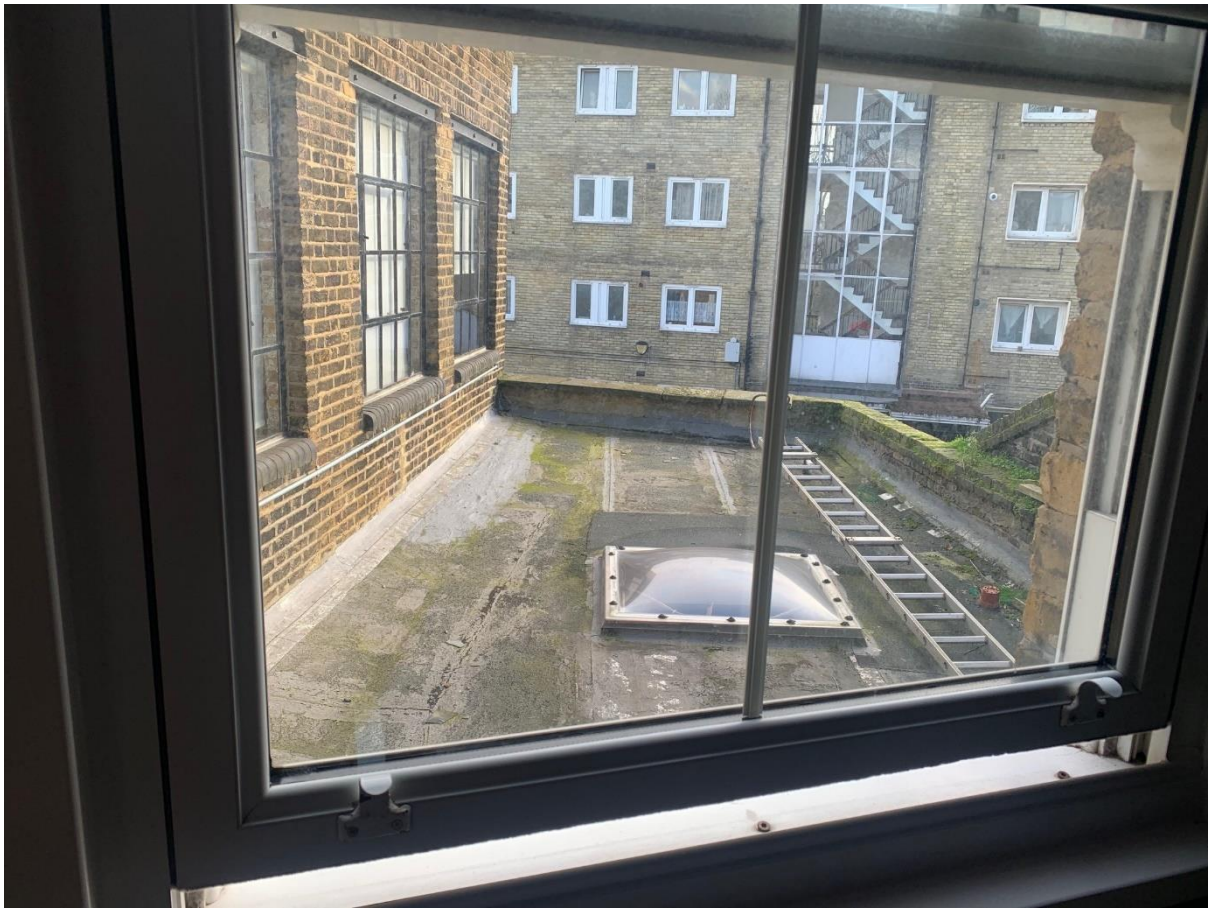
Rear extension view from upstairs flat window
