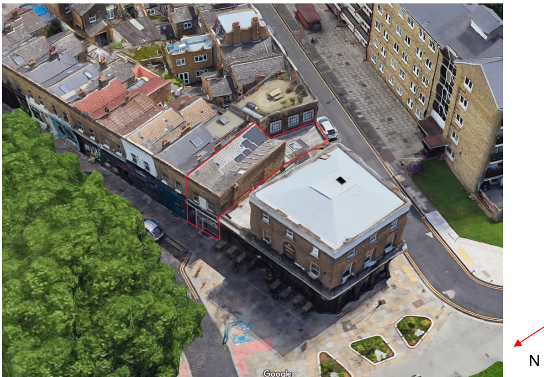
Figure 1 – Aerial photograph of the Site, viewing the Columbia Road shopping frontage with the Bird Cage Public House on the corner.
